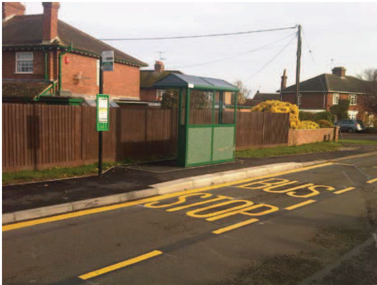
Figure 8.1: An example of an improved bus stop in Kintbury featuring new shelter, Kassel kerbing, pole and clearway.
